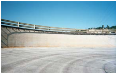
Clarifier after 6 years of liner service
