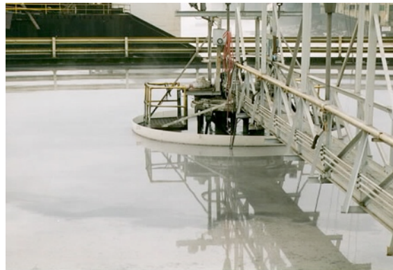
Wastewater Treatment Clarifier Coated with DuraShield 310
