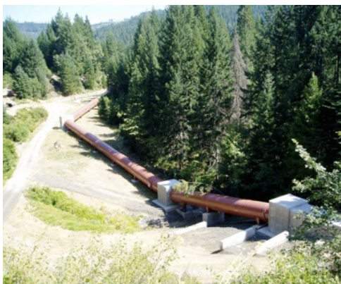
Completed Above-Ground 78" Welded Steel Pipeline
