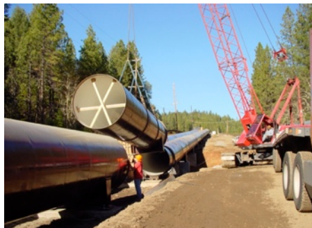
78" Welded Steel Pipe Installation
