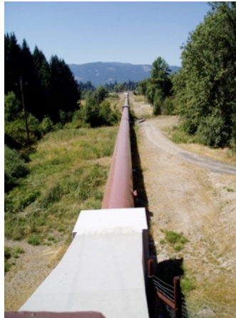
Penstock Pipe Heading to the Powerhouse
