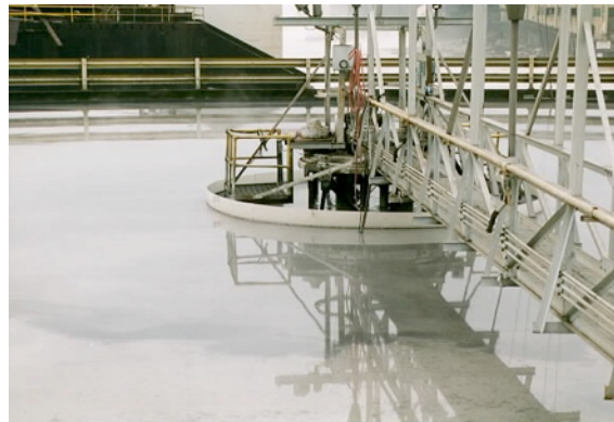
Wastewater Treatment Clarifier Coated with DuraShield 310
