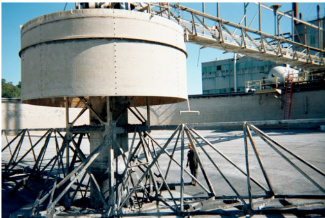
Clarifier Fill Tube 5 Year Inspection
