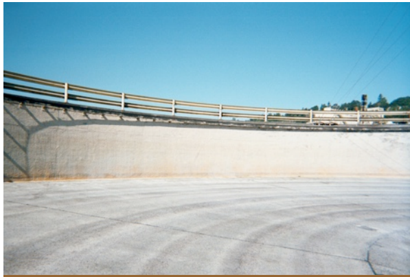
Wastewater Treatment Clarifier Empty During 5 Year Inspection of DuraShield 310 Coating
