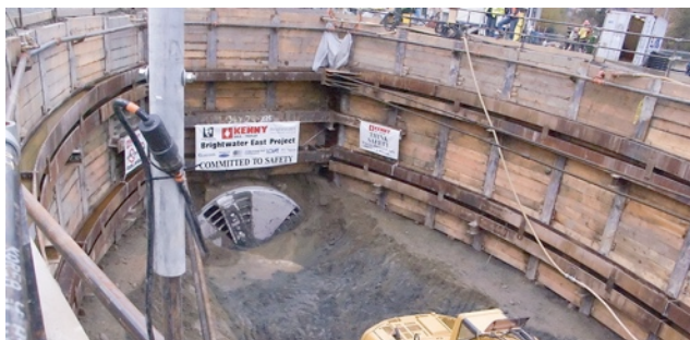
The Massive TBM Breaks Through
