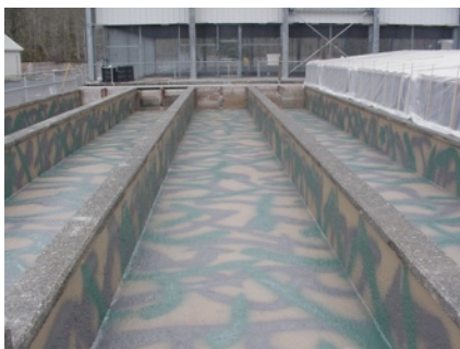
Raceway Coated with DuraShield 310-61
