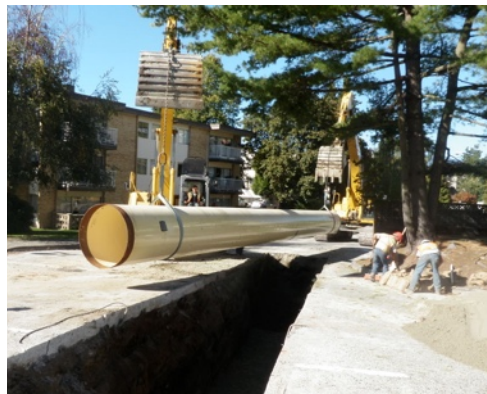
Crews install polyurethane coated steel pipe
