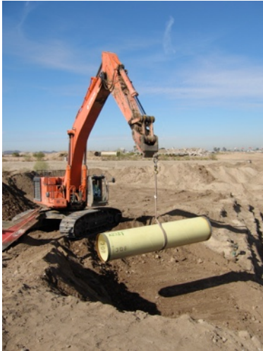
42" Welded Steel Pipe Installation
