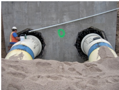
In Field Joint Coating with Heat Shrink Sleeves
