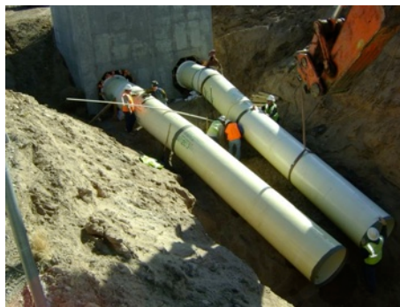
Twin Siphon 42" Welded Steel Pipe with DuraShield 210 Lining and Coating
