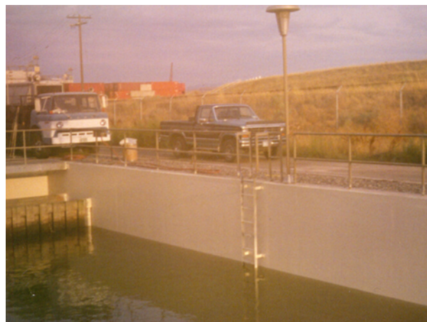
Chlorine Basin After Rehabilitation
